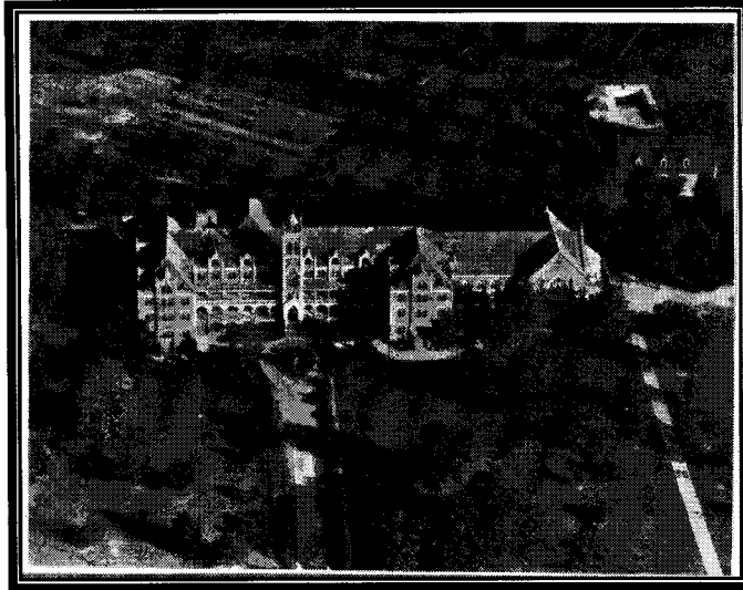
Aerial view of the school.
